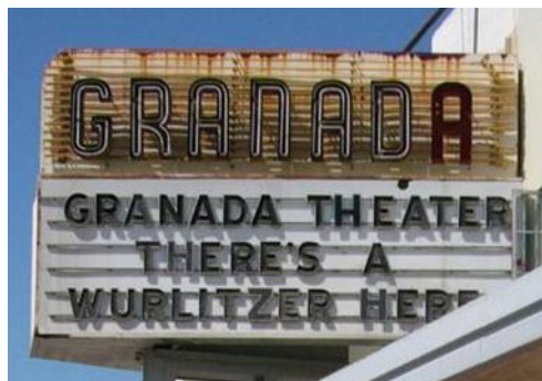
The Granada Theatre façade is typical of neighborhood movie houses across the country before TV ruled our lives. Photo by Gordon Bachlund
