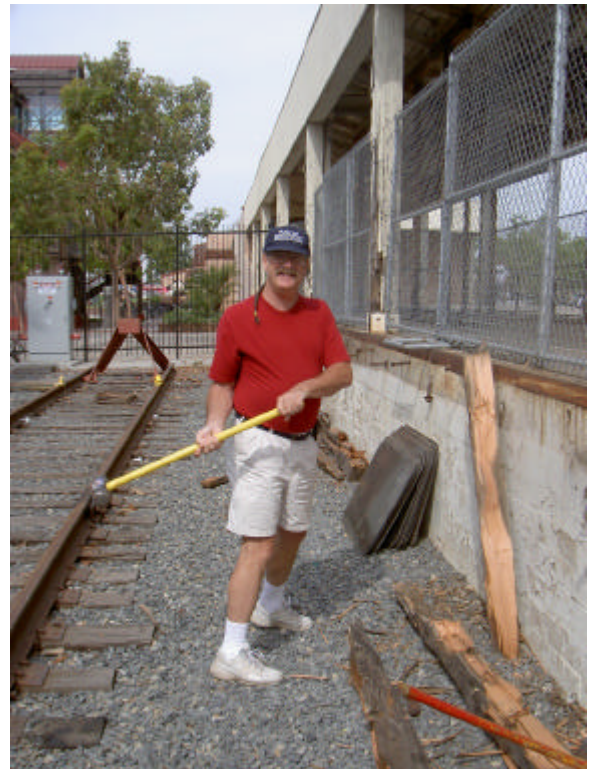
Jeff Schulze found that hitting the rotten bumpers with a sledge seemed to work well. Photo by Jack Barich
