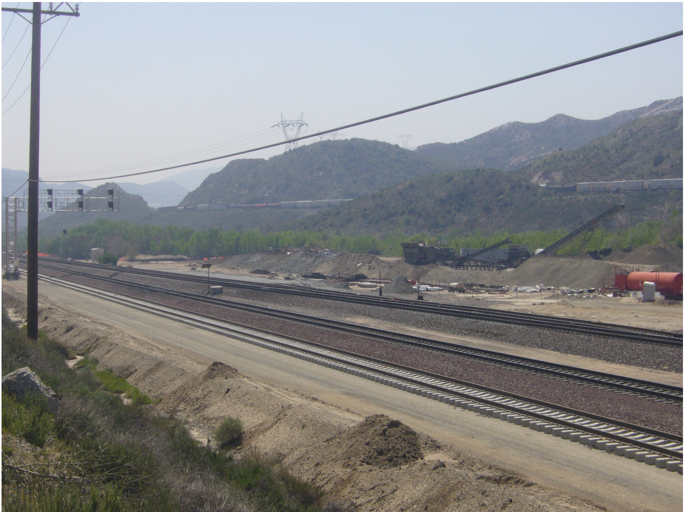
Above: New track on cement ties awaits the addition of ballast at Cajon. Note the new cantilever signal bridge spanning all three tracks. These new bridges, made of tubular steel, are replacing the more conventional block signals on bridges and staffs throughout the Southern California District of BNSF. Visible in the upper portion of the photo is an eastbound (timetable direction) Union Pacific freight heading down hill toward West Colton Yard. Photo on left: Looking east at Power Line Road toward Summit, four tracks are visible. Left to right, they are the Union Pacific Colton Cutoff (the uppermost track traveling from upper left hand corner to right hand corner); BNSF's new Track 1; BNSF Track 2 (1913 alignment) and BNSF Track 3 (1889 alignment). The photographer is standing on a knoll between the 1889 and 1913 alignment, a favorite place to watch trains.
