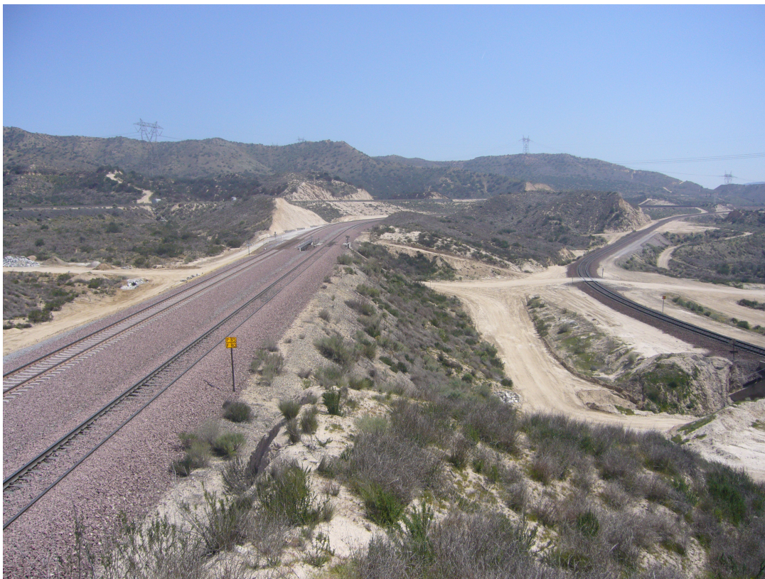
Above: New track on cement ties awaits the addition of ballast at Cajon. Note the new cantilever signal bridge spanning all three tracks. These new bridges, made of tubular steel, are replacing the more conventional block signals on bridges and staffs throughout the Southern California District of BNSF. Visible in the upper portion of the photo is an eastbound (timetable direction) Union Pacific freight heading down hill toward West Colton Yard. Photo on left: Looking east at Power Line Road toward Summit, four tracks are visible. Left to right, they are the Union Pacific Colton Cutoff (the uppermost track traveling from upper left hand corner to right hand corner); BNSF's new Track 1; BNSF Track 2 (1913 alignment) and BNSF Track 3 (1889 alignment). The photographer is standing on a knoll between the 1889 and 1913 alignment, a favorite place to watch trains.
