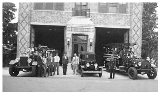
The Wilshire building, opened in 1926, served double-duty as firehouse and City Hall. Photos © Fullerton Public Library
